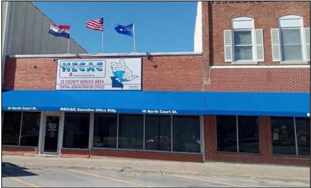
Central Administration Executive Office Building 16 N. Court, Bowling Green, Mo., 63334 1-800-748-7636
