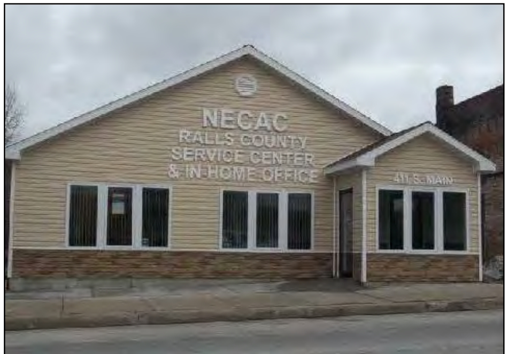
Ralls County Service Center 411 Main in New London 573-985-2411
