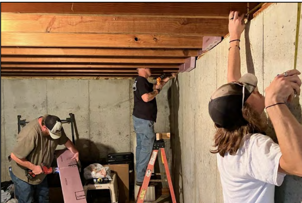
Upgrades provided by NECAC Weatherization Crew Members Jacob Schler, left, Kenny Chastain and Zach Kilby will mean greater energy savings for the client.
