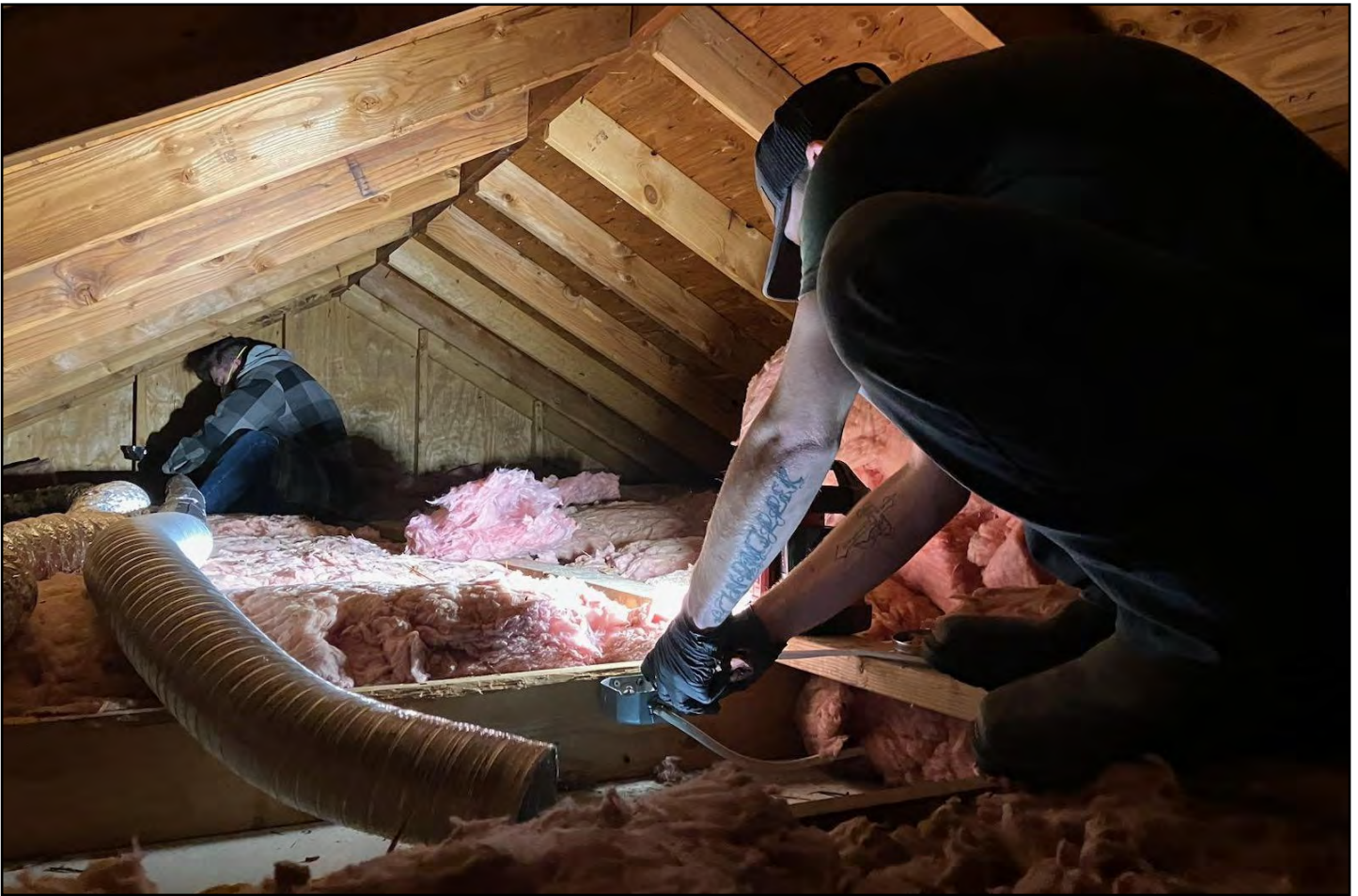
NECAC Weatherization Crew Members Zaqry Uplinger, left, and Jacob Windmiller insulate an attic.
