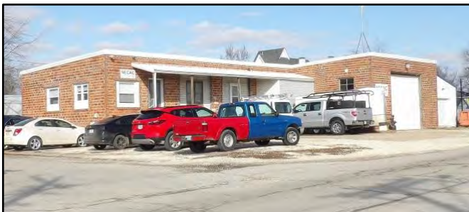
Weatherization Warehouse 619 E. Champ Clark Drive, Bowling Green, Mo., 63334 573-324-2251
